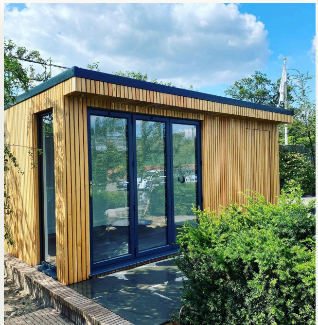
...TO THE FINISHED SPACE
